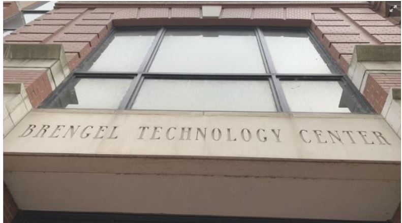
The Brengel Technology Center at 507 E. Michigan St. in downtown Milwaukee is on the block that could be sold to Bear Real Estate. - NICK WILLIAMS
